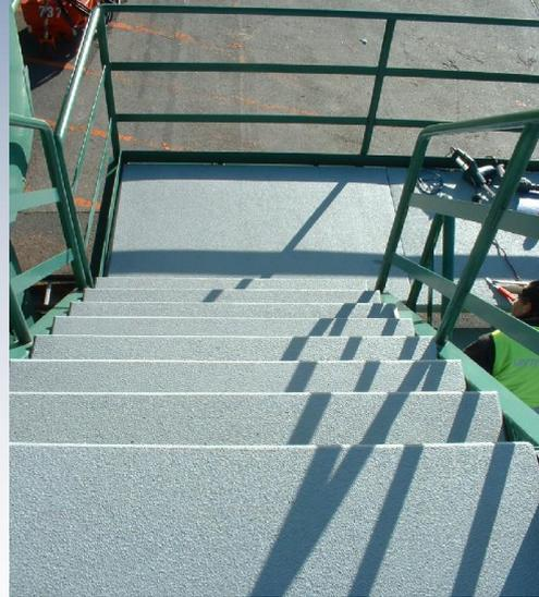
Boarding stairway with smooth anti-skid surface and integrated heating function from SwedeSafe.
